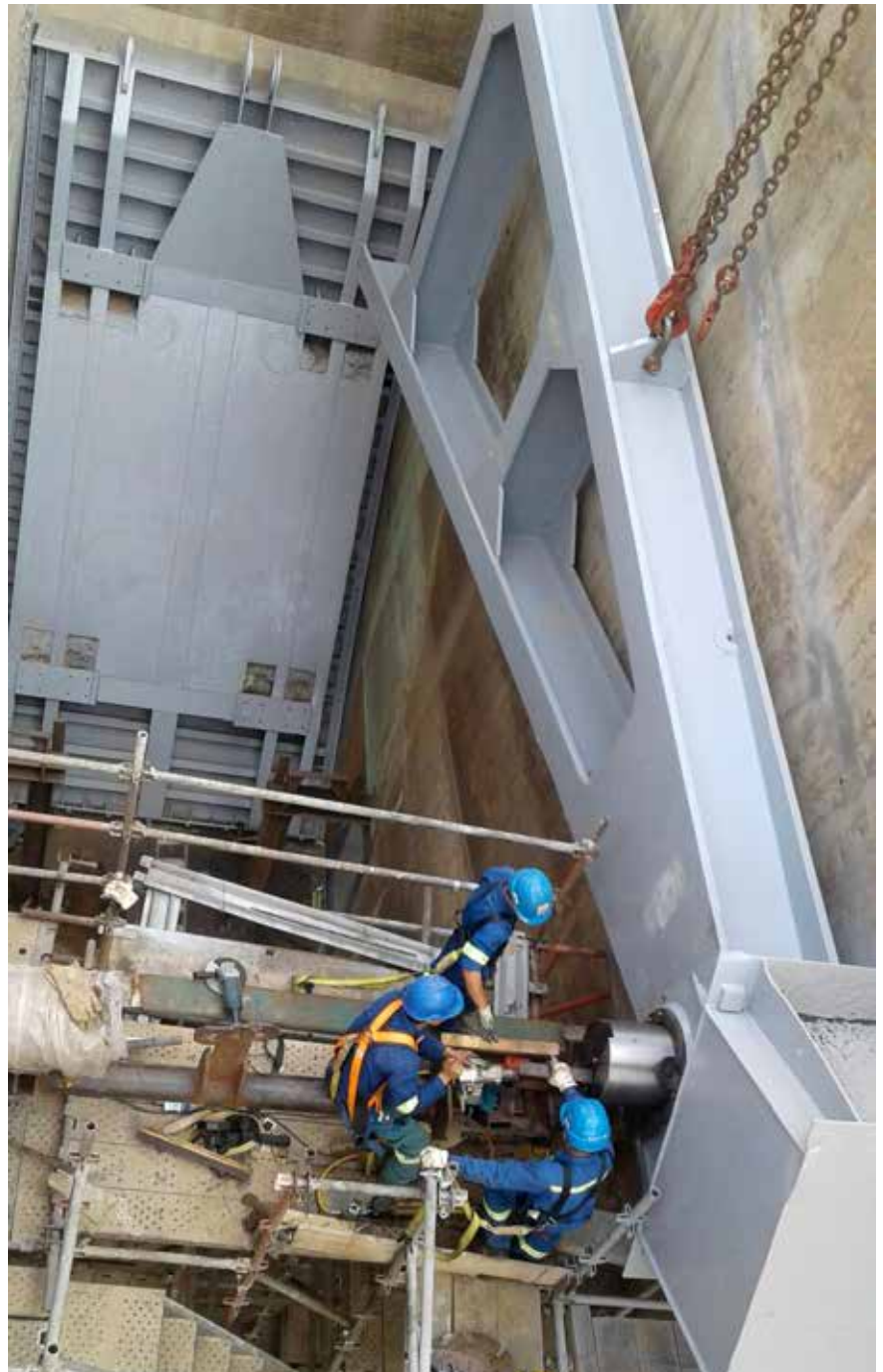
Mounting the arms of the radial gates
