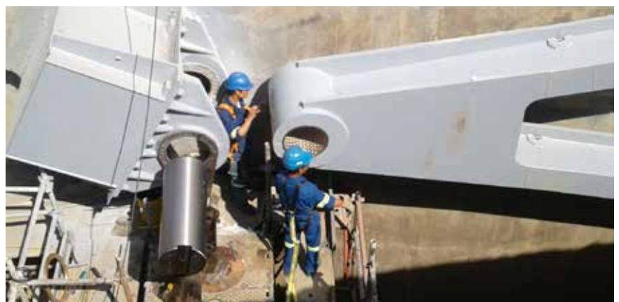
Mounting the arms of the radial gates
