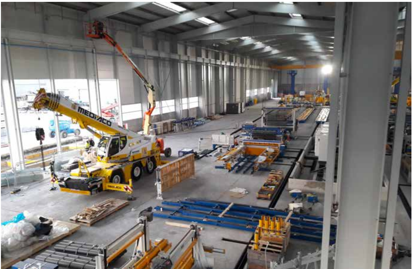
Montereau - (France): Construction of the "Atelier treillisoudes"
