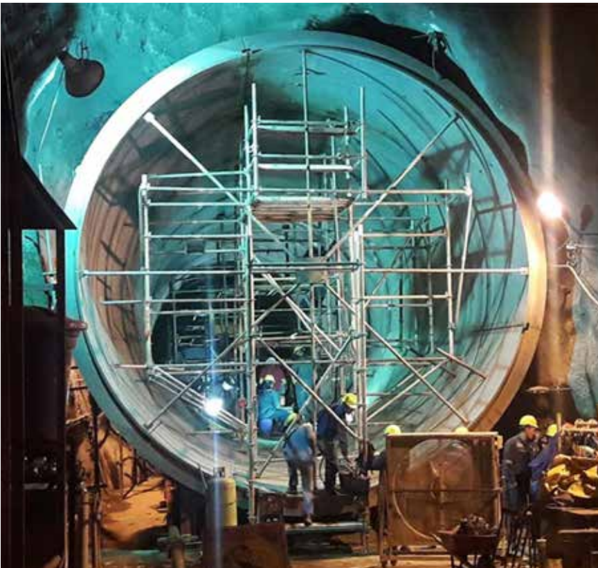
The Ituango worksite
