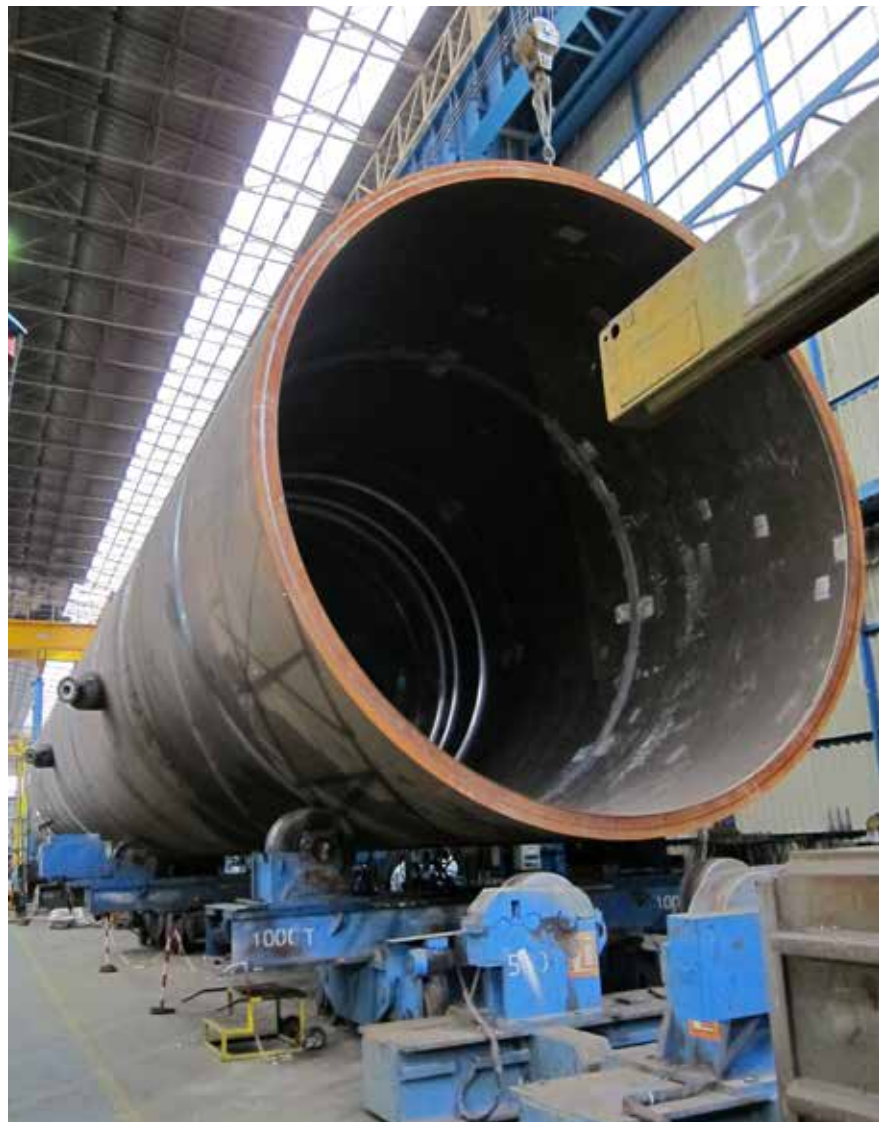
The assembly stages in the Porto Marghera plant, Venice.
