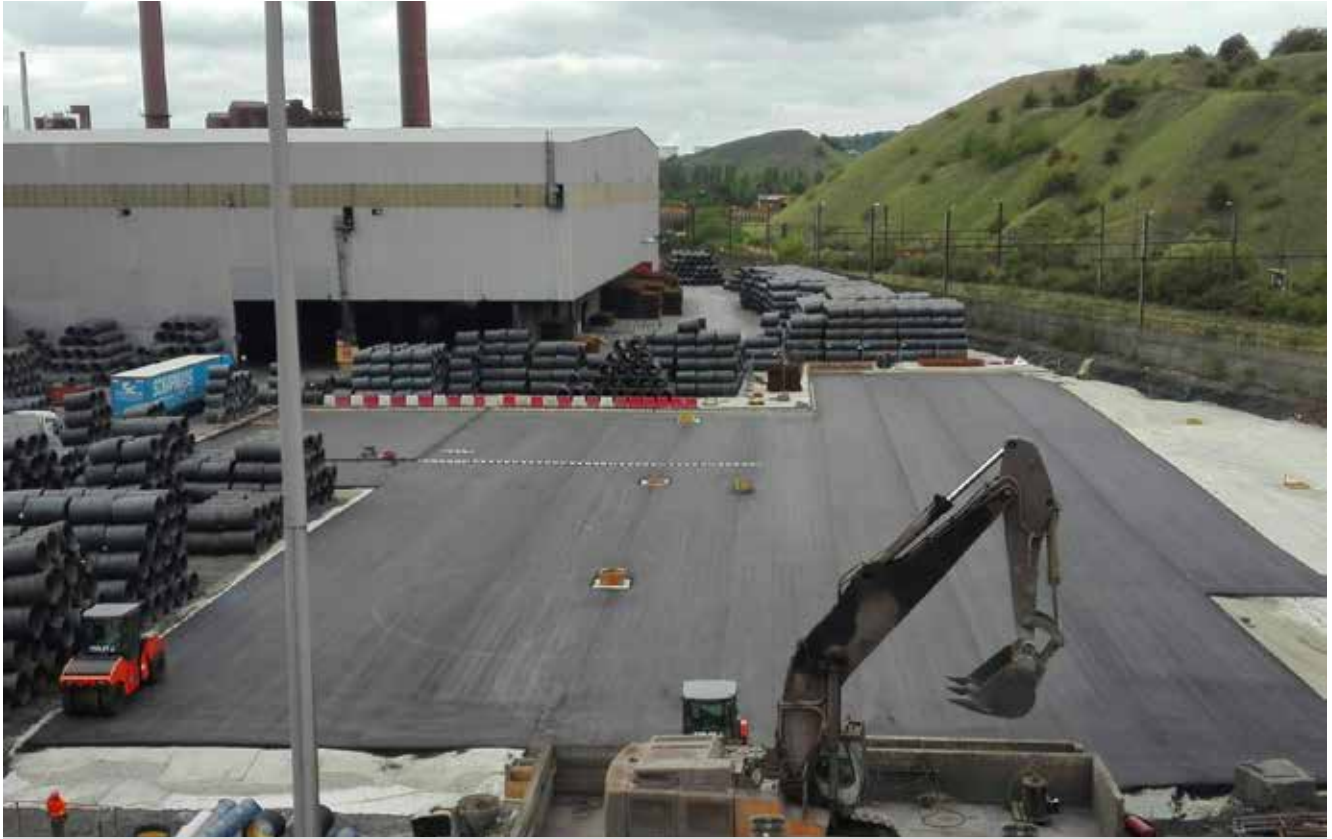
Thy Marcinelle - (Belgium): Construction of the flooring for coil storage
